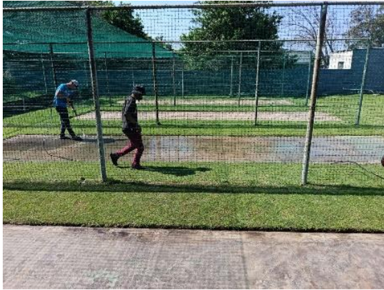
Cricket nets revamp in progress.
